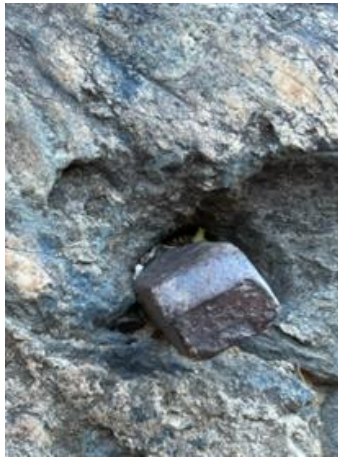
Over 200-year-old iron wedge stuck in the lock wall.
