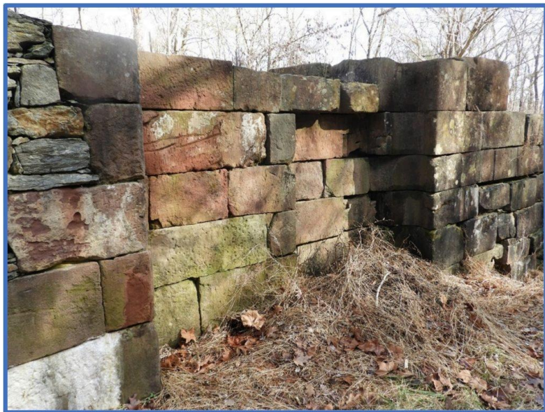
Close-up of Lock 2. It is constructed of red sandstone, which was available at the Seneca sandstone quarry just 10 miles up-river.
