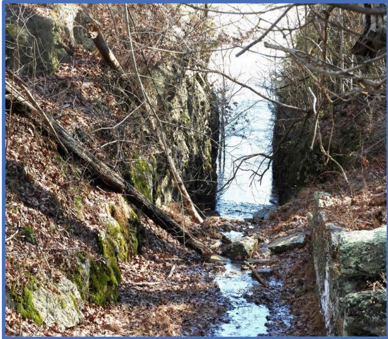
A cut through metamorphic rock for Locks 3, 4, and 5.
